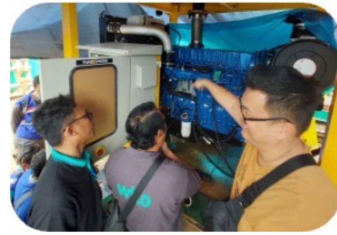
On site commission training
